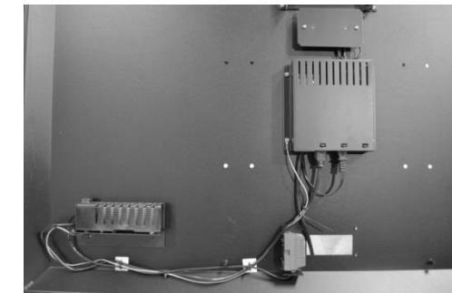
**IMPORTANT!** Carefully follow the layout on the applicable photo for your enclosure and TV to ensure that the heater and wire harness will not interfere with the enclosure Z-brackets and the thermostat will be accessible from the cable cover opening for future adjustments. **Use Extension Ground Wire for AE6560 – see Grounding**
