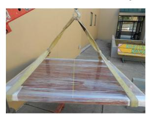
Remove the packaging from the first top half and install net with three 3/8" flathead bolts.
