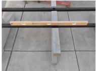
Level table by placing shims under legs if needed.
