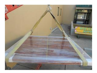
To place the table top halves the threaded insets should be orientated down (as shipped). The threaded insets for the net installation orientate towards the center of the table (middle leg). Placing table tops is best done using 12' lifting straps and forklift, tractor or boom truck. Place table halves with packaging wrap in place to avoid damaging the concrete. Two men should make manual adjustments to align the bolt holes under the slab with the threads on the underside of table top.
